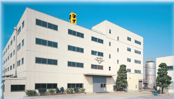
Osaka Plant (CT, Wear Parts)
